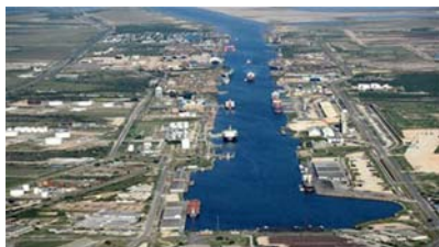
Port of Brownsville Shipping Channel
